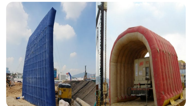
Installation Site of Inflatable Soundproof Barriers for Noise Management
